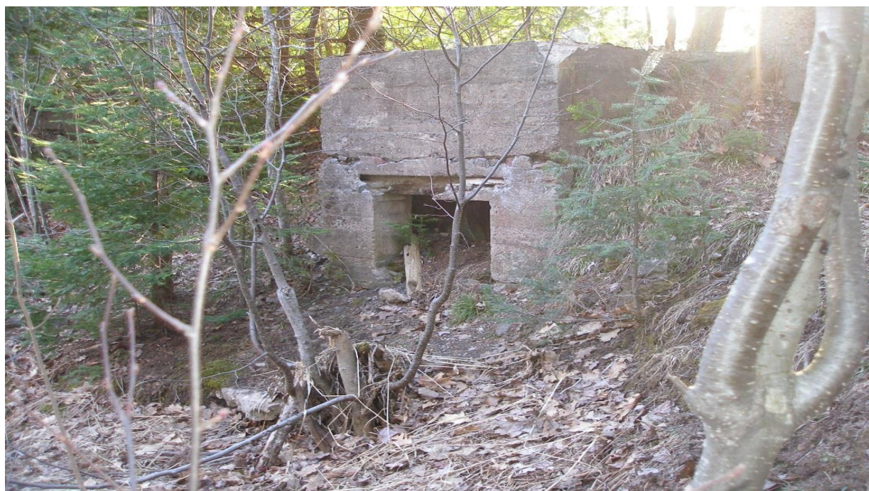
Photo 1. The water intake of the Finnish Farmers Milling Company grist mill on the Boston Creek, August 2016. It is the largest structure that can still be seen. The view is to the south. To the left is the broken-down dam which is barely visible. Photo by Dana Richter.
