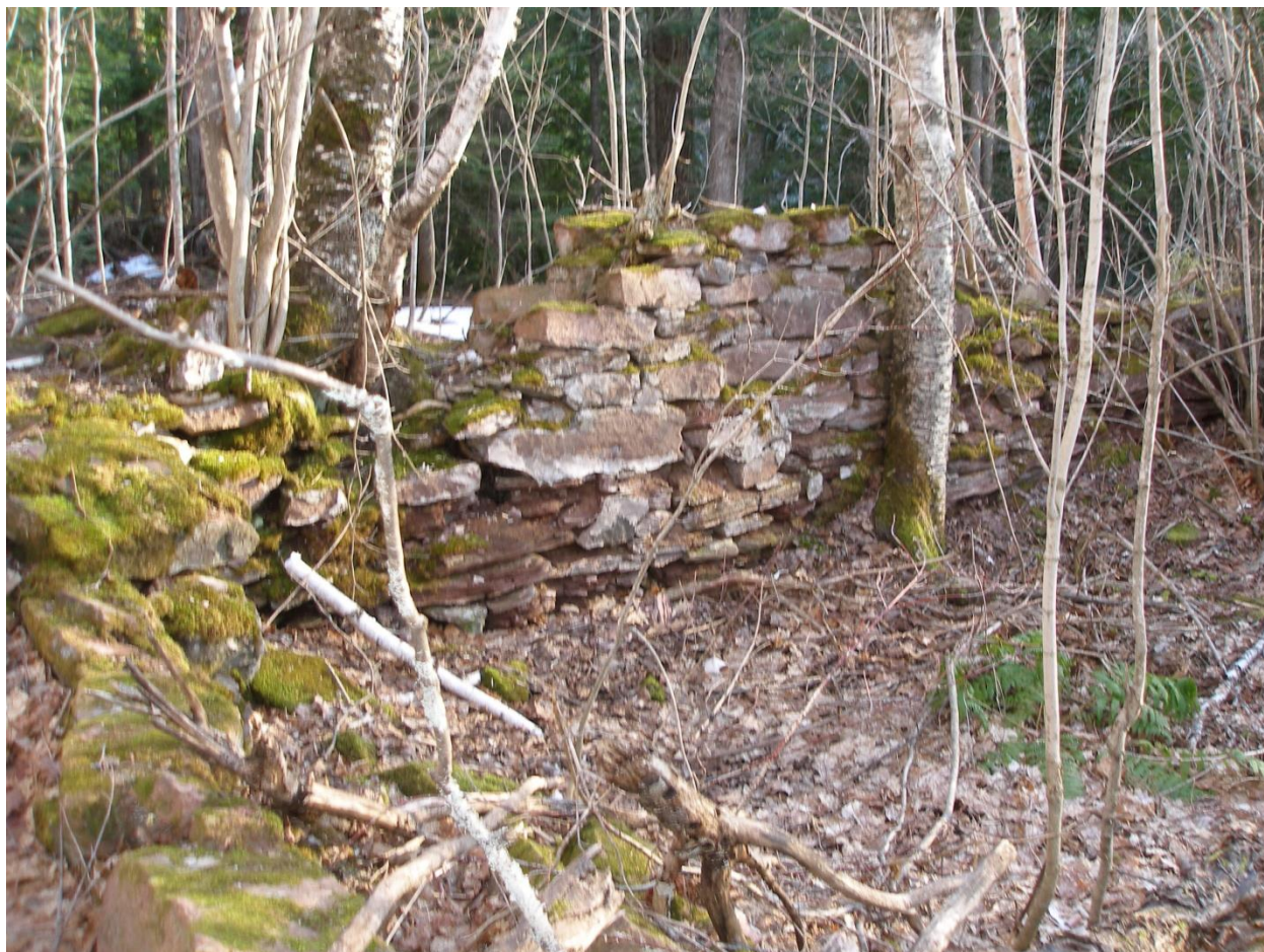
Photo 3. Mostly sandstone foundation of the grist mill that lies approximately 225 yards (0.13 mi) downstream from the dam on the Boston Creek. View is from the west; the Boston Creek flows approx. 100 ft below and 20 ft beyond the foundation. Photo by Dana Richter.
