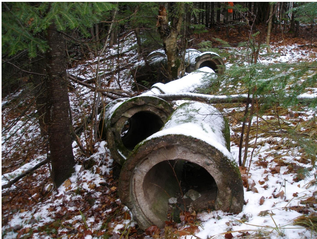
Photo 2. Part of the concrete piping of the Finnish Farmers Milling Company on the Boston Creek that brought water from the dam intake to the water wheel that ground grain to make flour or feed. View is to the west; to the left is Boston Creek. Photo by Dana Richter.
